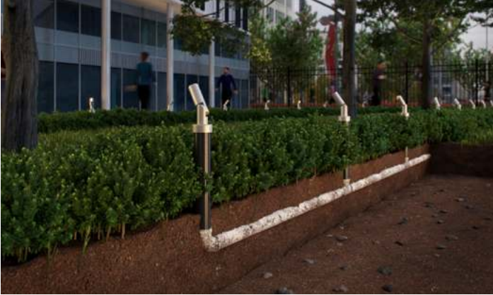
L930 B2 | Landscape | During Installation
