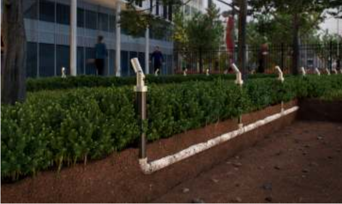
L930 B2 | Landscape | During Installation
