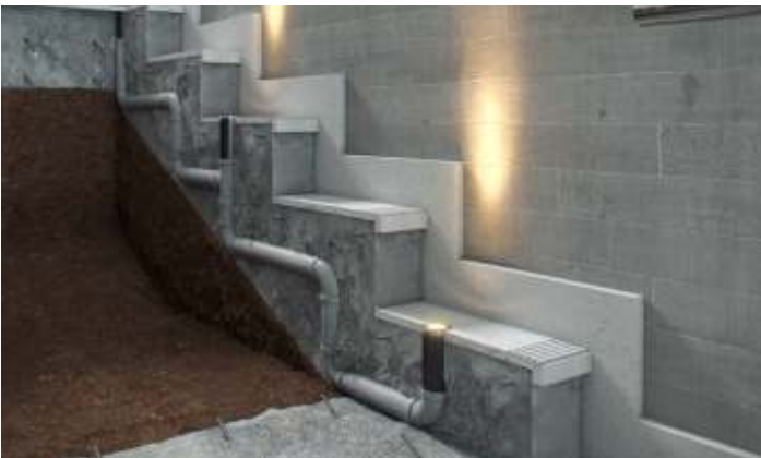
L01 | Stairs/Ground | During Installation
